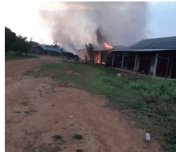
Damage to the Basic Education Primary School in Talan Zar Village, Falam Township, Chin State, following a military airstrike on 4 May 2026.
